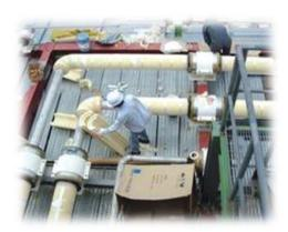
**TIC Bwrap** is wrapping foam of product symbolized protection from external conditions. Vapor Barrier, wrapping type of self adhesive products, convenient to use at construction site and excellent performance to resist moisture blocking at the steam plant.
